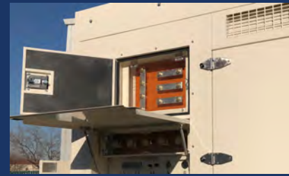
LINK BOARD VOLTAGE SELECTION
